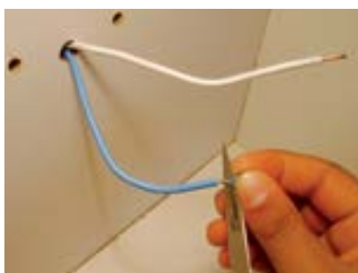
10. Descapcar as pontas dos fios (1cm).
