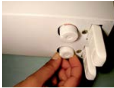
49. Colocar os starters nos porta starters.
